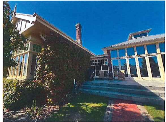
Figure 3 - View of 4 Norwood Avenue, showing new design (extension) in old setting
