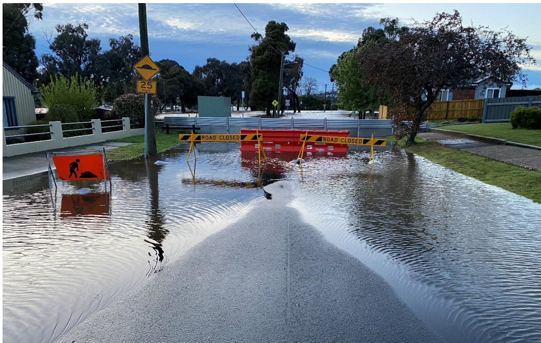
Hart St Gate (NG1) leaking during October 2022 Flood
