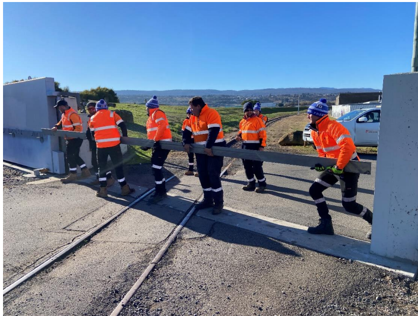
Closure of the Glebe Farm Gate (EG1). The length and weight of this log is of concern and is planned for rectification
