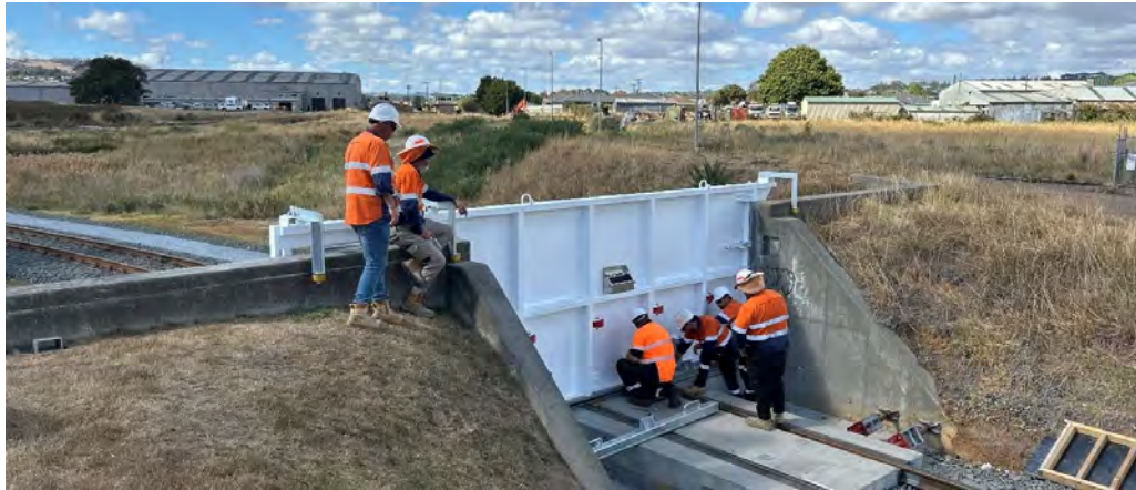
Figure 1 - Edilon Sedra slabtrack in position beneath levee gate EG2.
