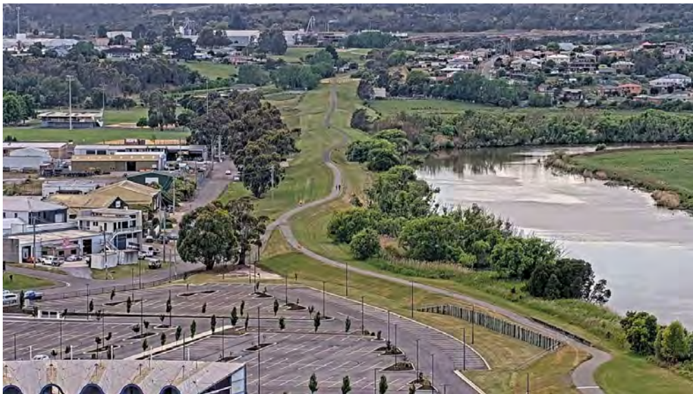
Figure 6 - Invermay Levee from UTAS Stadium Camera.
