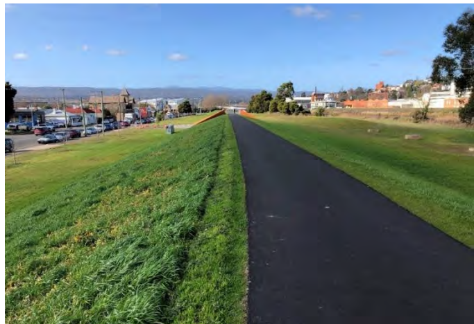
Figure 2 - View along levee crest toward Tamar Street
