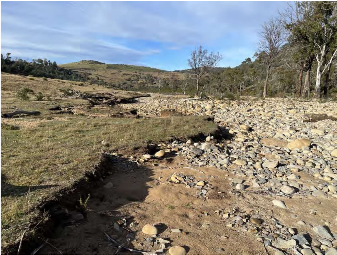
Figure A4-7: Evidence of previous water erosion from past flood events along the banks of the North Esk.
