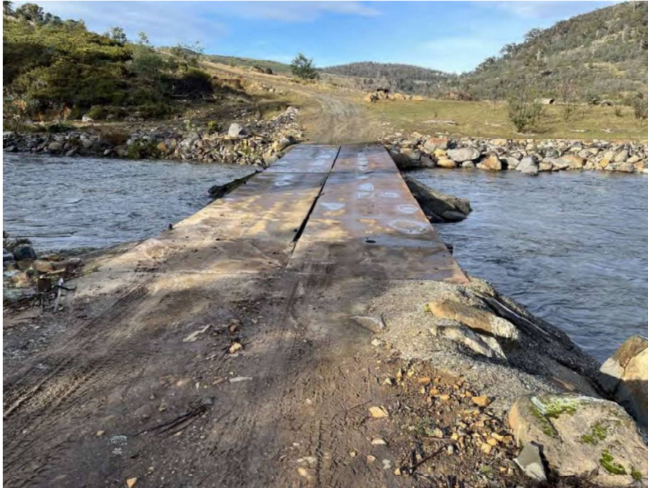
Figure A4-5: Existing bridge over the North Esk River that connects the property titles.
