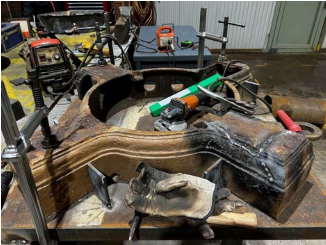
Figure 92 Photo showing base repair underway, note that the far side locating pocket for the fountain body is broken
