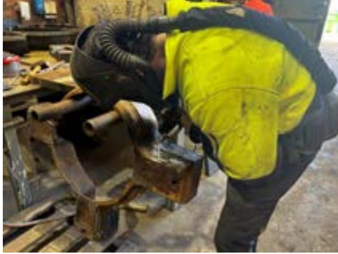
Figure 82a Photo showing base repair underway
