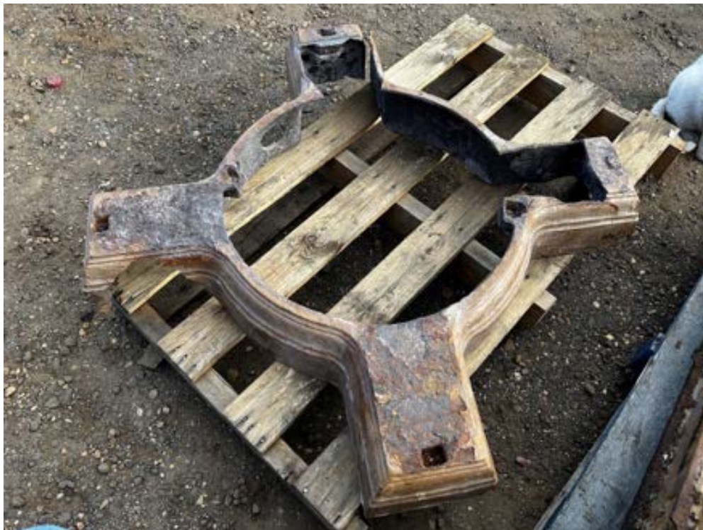
Figure 91 Photo showing the poor condition of the fountain base
