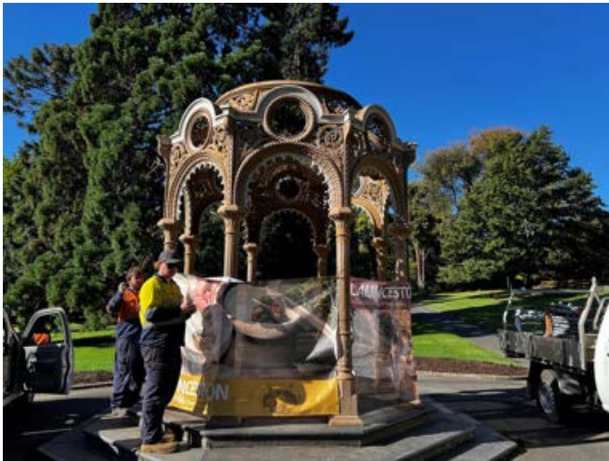
Figure 24 Photo showing dome removed
