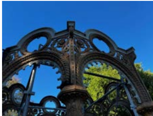
Figure 32 Showing Corbel Cover Plates in Position
