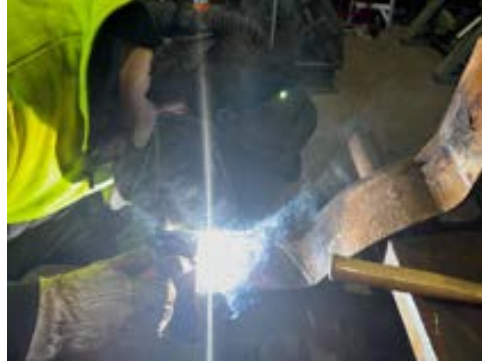
Figure 82b Photo showing base repair underway
