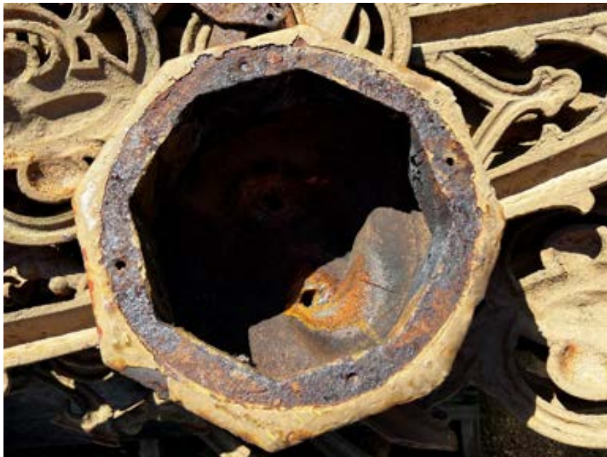
Figure 22 Showing the underside of the crown, the four retaining bolt holes for the Sun Casting on the underside are visible
