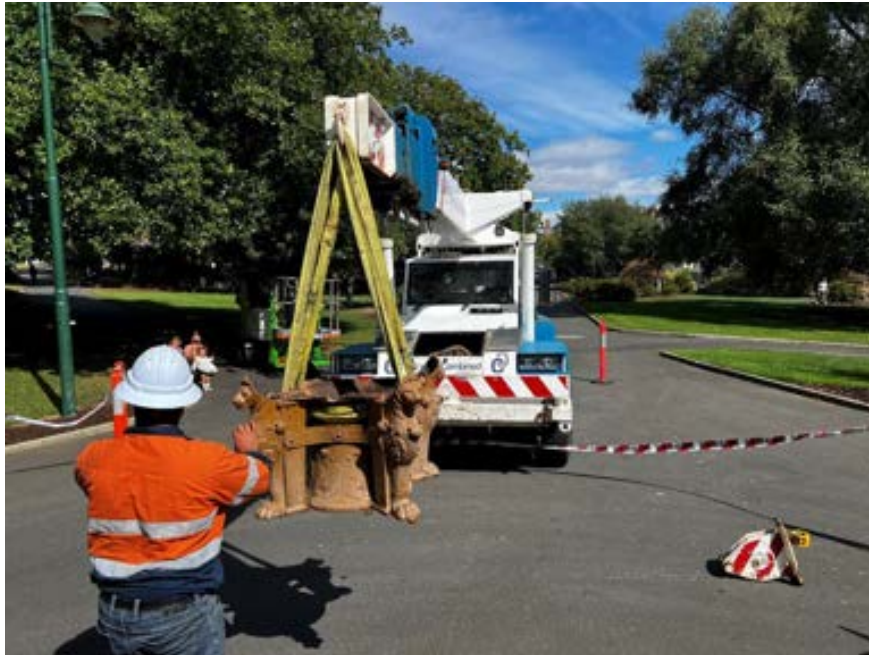
Figure 6 Shows the bowl support being removed
