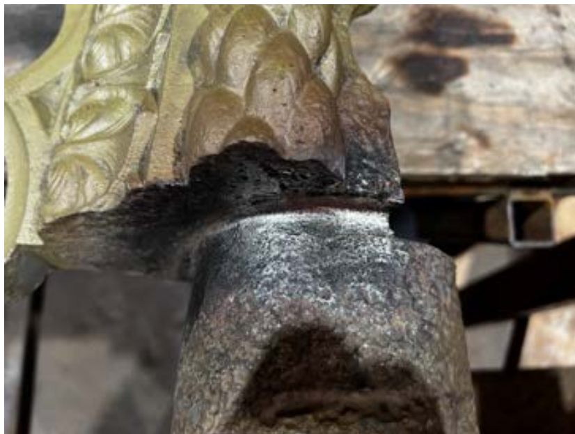
Figure 108 Photo showing completed and dressed weld repair
