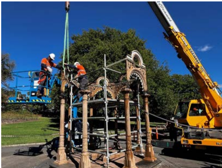
Figure 43 Removing the cusped arch face panels
