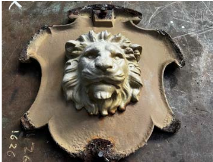
Figure 13 Showing internal section of the Memorial Shield with the lion mascaron, all the shields have lion mascarons attached internally and four different designs externally this one stating "Erected on Her Majesty's Diamond Jubilee 20 th June 1897 You can see the heat marks and retaining bolts cut off
