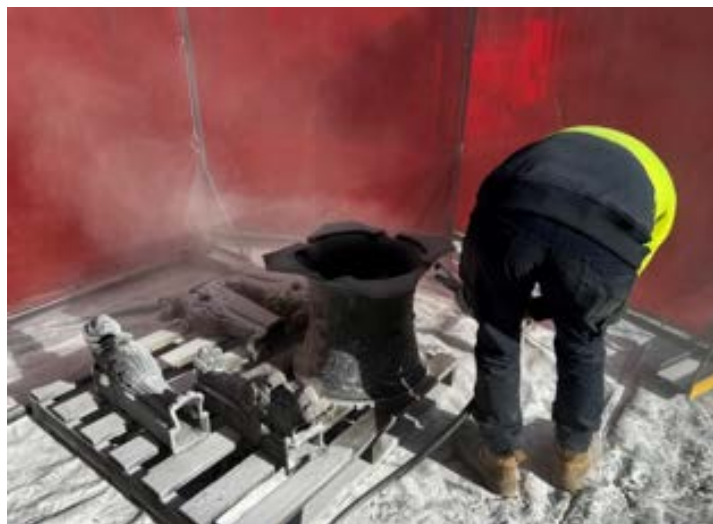
Figure 62 Photo showing dry soda blasting underway
