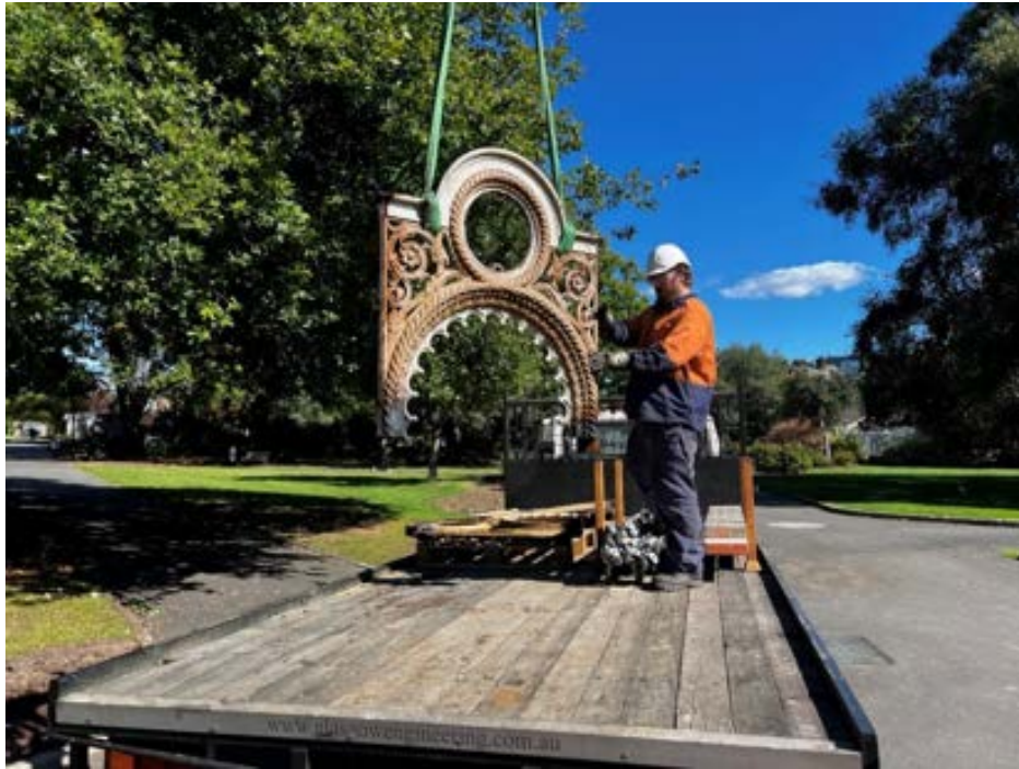
Figure 42 Photo showing one of the four intact cusped arch face panels being removed
