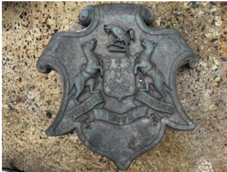
Figure 59 Shows the beautiful cast details in the shield after paint stripping and wet soda blasting
