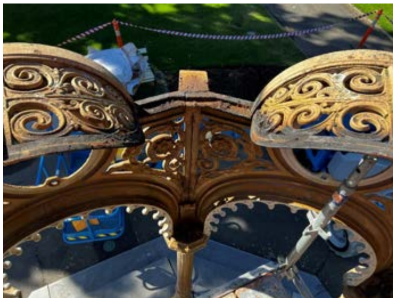
Figure 25 Photo showing pendentive being removed with heat and drilling
