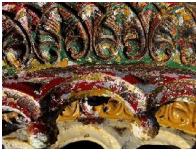
Figure 60 Photo showing the plethora of colours painted over the years. Some of the previous colour schemes we uncovered that were painted over the original were Post Box Red with Yellow highlights, Brunswick Green and Gold painted highlights, Silver Frost all over luckily for the people of Launceston this only seemed to be one coat, a light Turquoise colour, many coats of pink primer, red & orange red lead undercoat and the current colours of X41Buff and X34 Driftwood with Y35 Off White highlights
