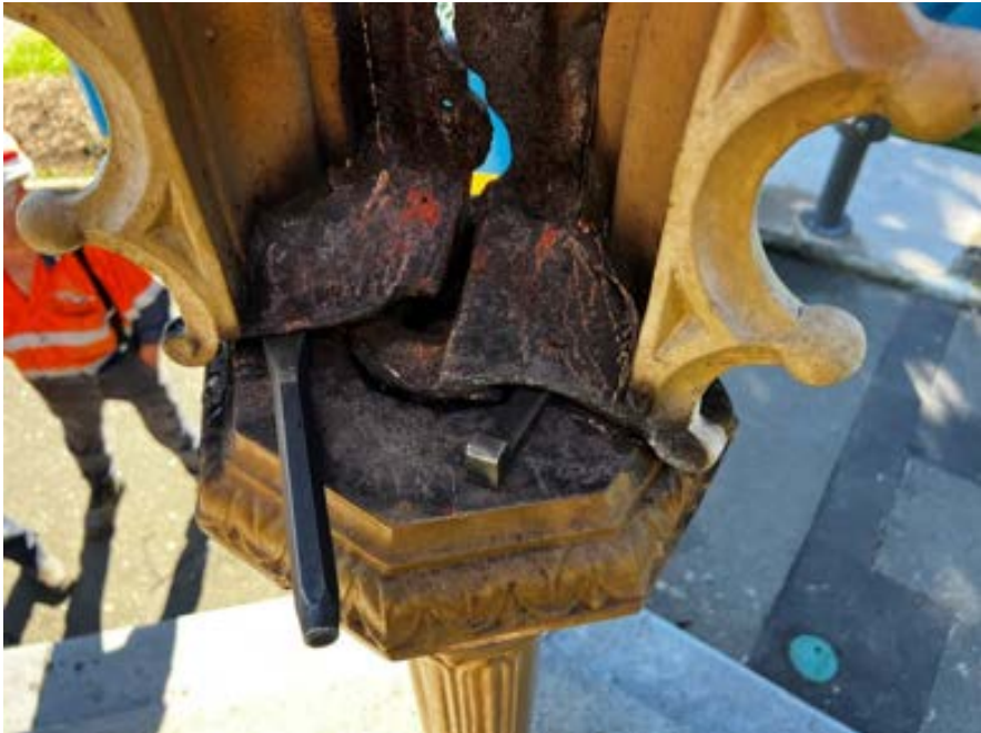
Figure 36 Shows us trying to wedge the plug out of the socket
