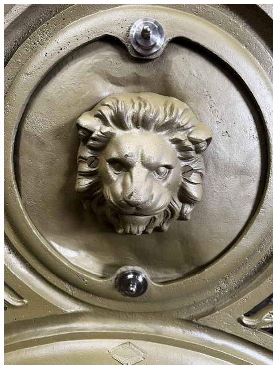
Figure 110 Photo showing before and after with new 316 stainless
