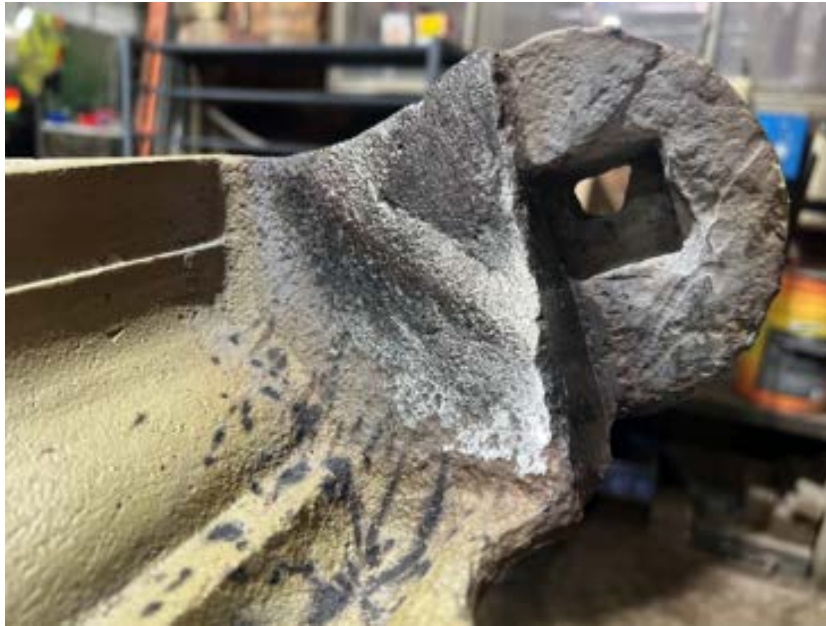
Figure 107 Photo showing completed and dressed weld repair
