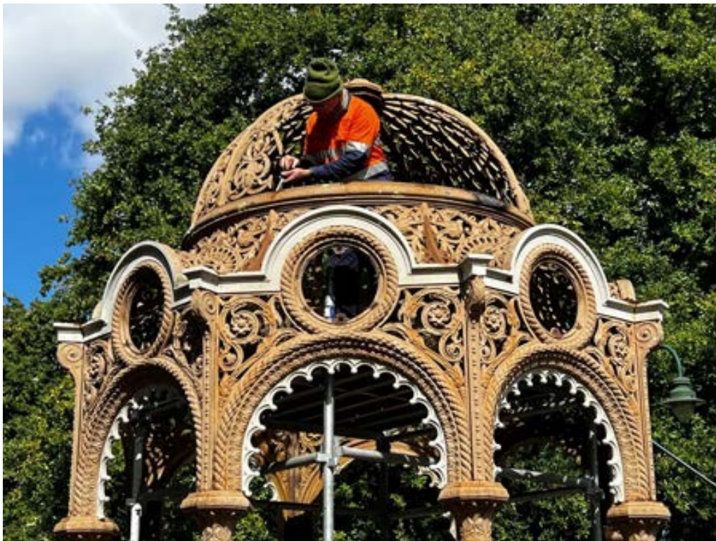
Figure 23 Photo showing removal of the cast filigree dome
