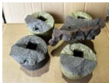
Figure 100 Photo showing the four broken face panel plugs
