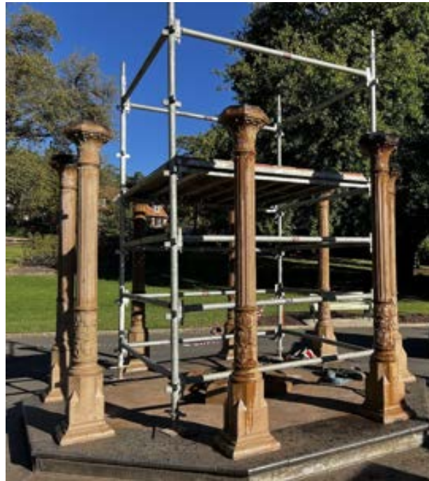
Figure 131 Photo showing the eight columns on site
