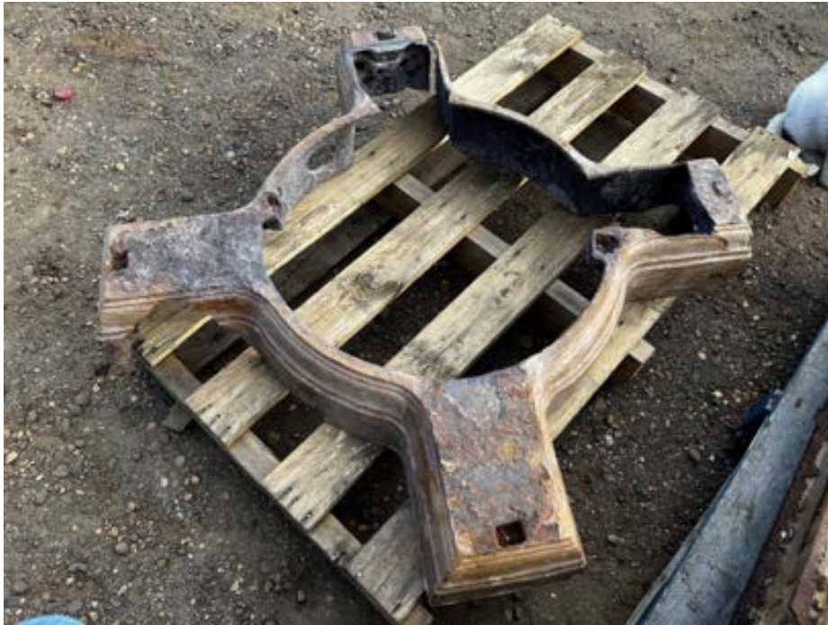
Figure 52 Photo showing the base removed with damages and corrosion
