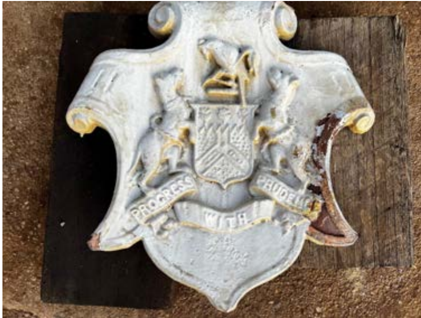
Figure 57 Photo showing the memorial shield as we were undertaking a little investigative work, carefully removing the layers of paint with a heat gun and scalpel, we revealed the original colour scheme under the many layers of paint.
