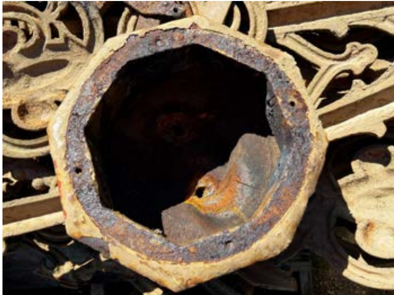
Figure 69 Photo showing the underside of the crown
