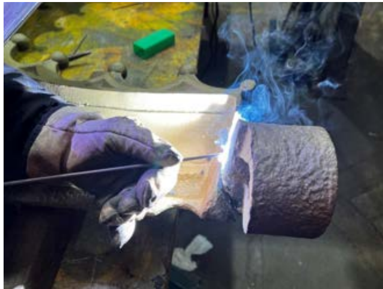
Figure 106 Photo showing plug being welded to the face panel
