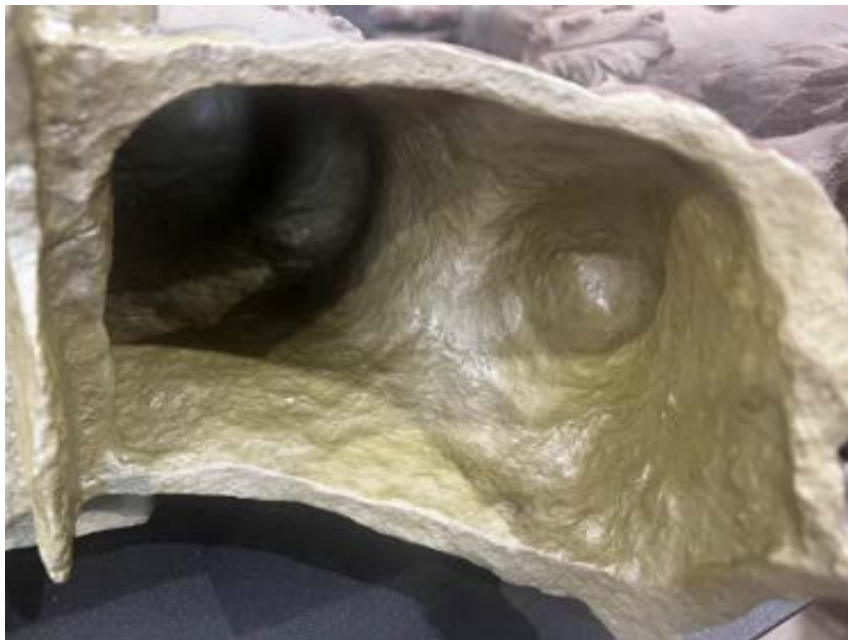
Figure 64 Photo showing the inside of the monopodia lion head bowl supports, these will have three coats of Sigma Prime internally to stop any further corrosion.
