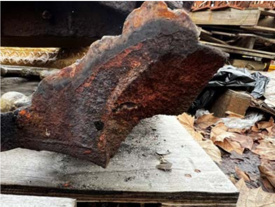
Figure 47 Shows number 4 of 4 broken sections on the Cusped Arch Front Face Panels where the plug attaches
