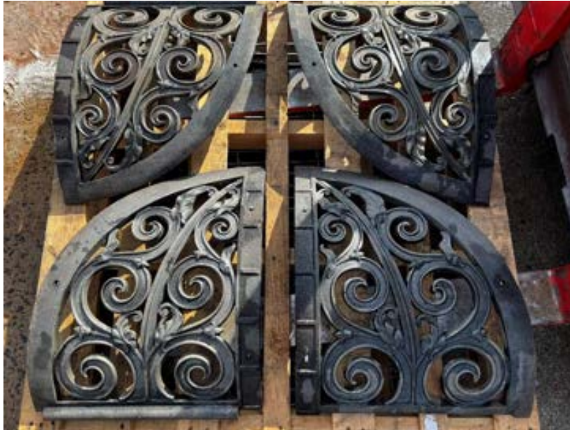
Figure 63 Photo showing parts of the pendentive after hand paint stripping and soda blasting
