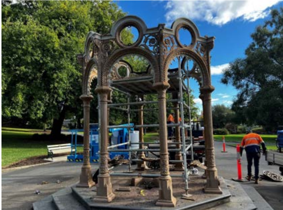
Figure 31 Photo showing the pendentive and lunette open cast filigree sections removed
