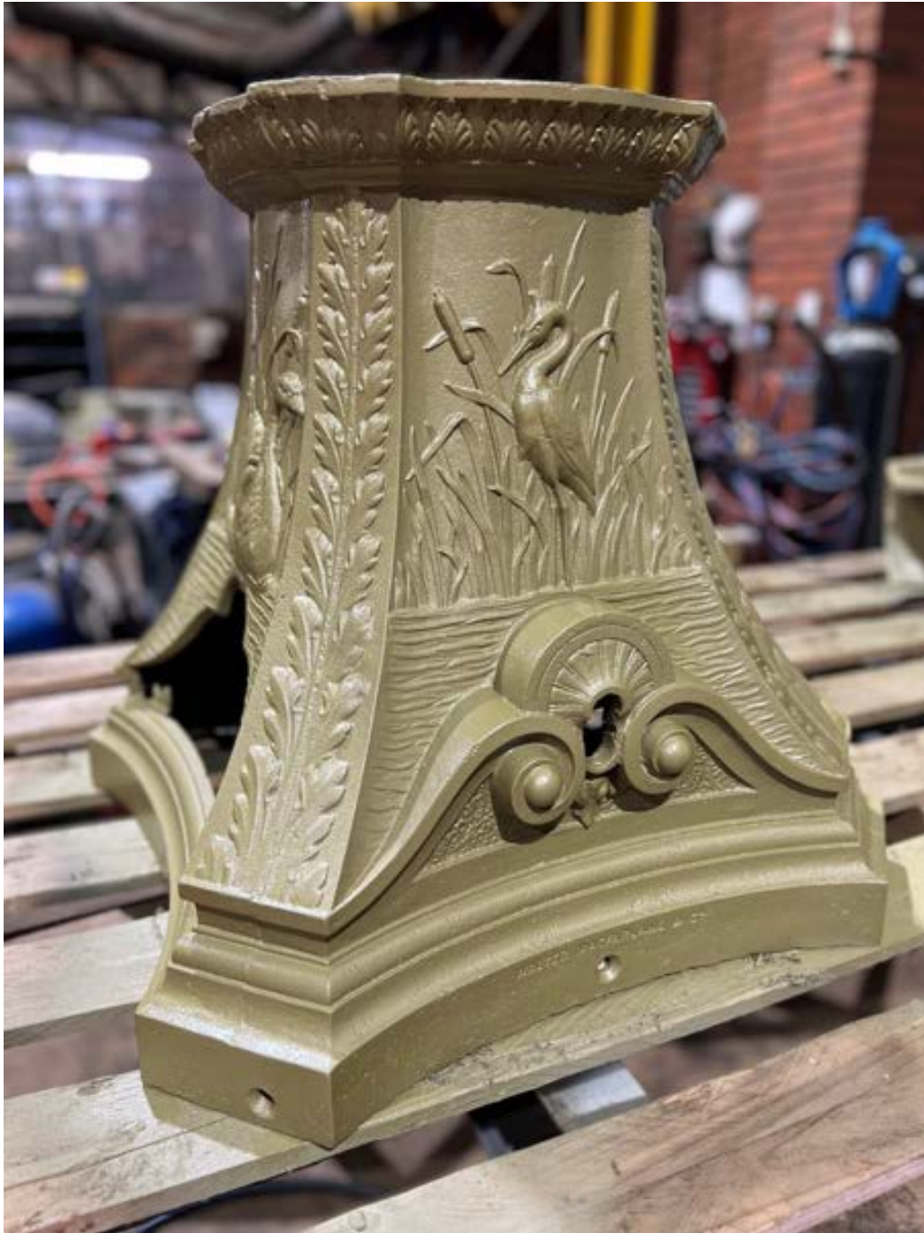
Figure 67 Photo showing the beautiful level of workmanship hidden by the many layers of paint. This level of casting is hard to match these days, its truly a credit to the patternmaker as all these reliefs would have been carved out by hand in timber first to make the pattern before the molten metal was poured.
