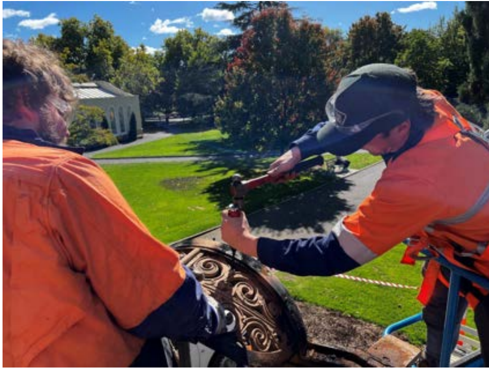
Figure 30 Removing the lunette open filigree sections
