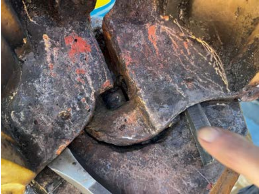
Figure 37 Show us driving wedges under the cast face panels
