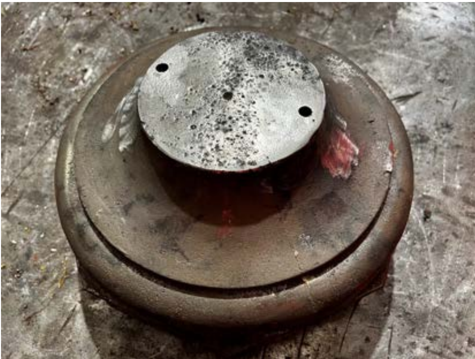
Figure 74 Photo showing the external repaired section of the dome
