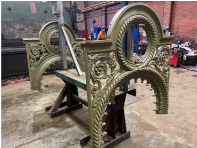
Figure 102 Photo showing front face panels being painted with Sigma Prime 200
