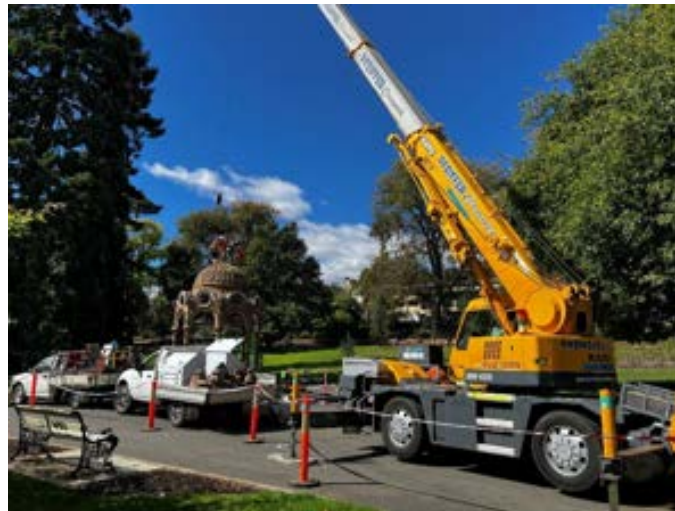
Figure 17 Showing removal of the eagle finial
