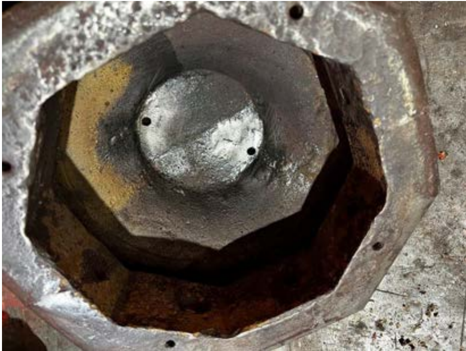
Figure 73 Photo showing the internal repaired section of the crown
