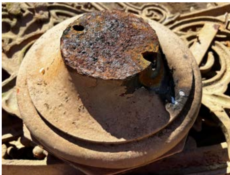
Figure 70 Photo showing the top side of the crown, visible on the right side is a small blow out section from using the oxy acetylene
