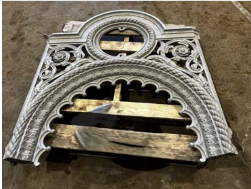
Figure 101 Photo showing lightly blasted front face panel
