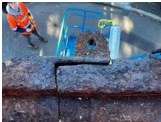
Figure 34 Shows Corbel retaining tab drilled out
