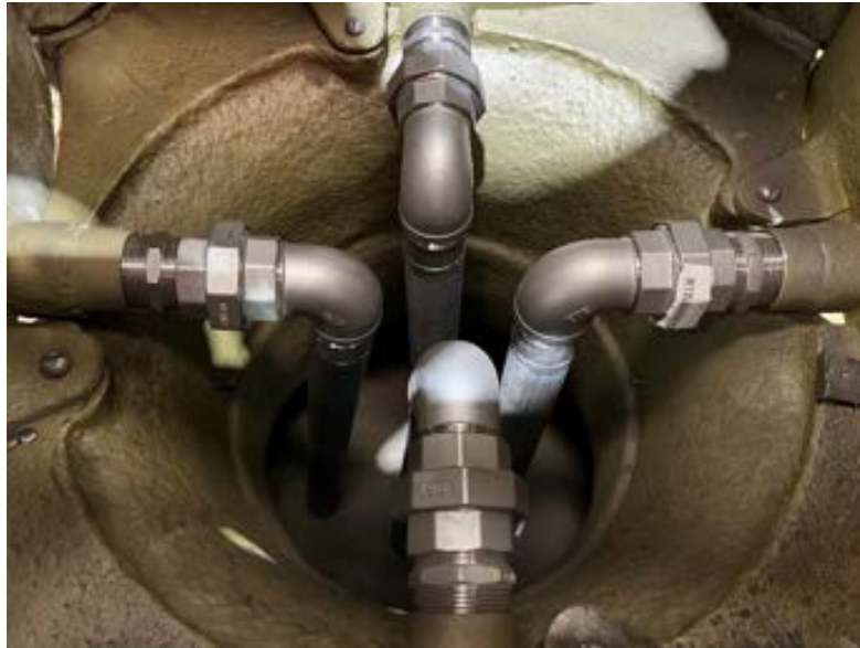
Figure 96 Photo showing new 316 stainless steel pipe work inside the fountain
