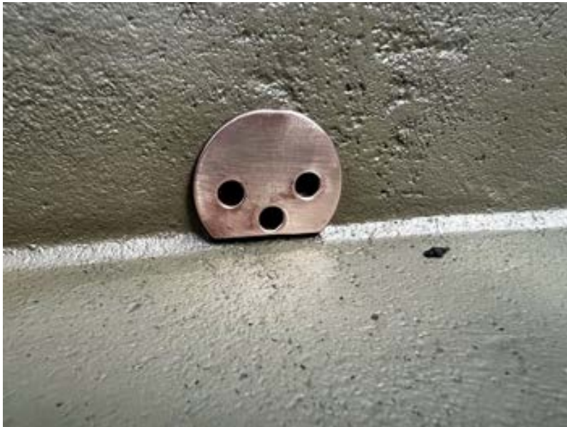
Figure 89 Photo showing new bronze cover plates bolted internally
