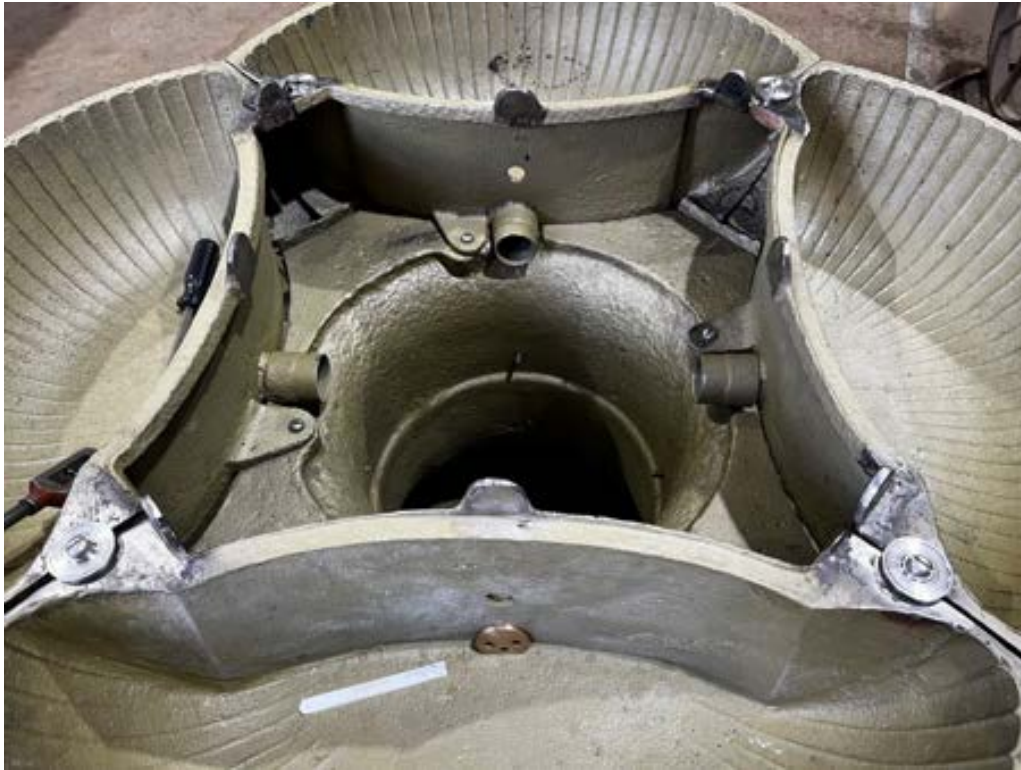
Figure 90 Photo showing four new 316 stainless steel drain sockets
