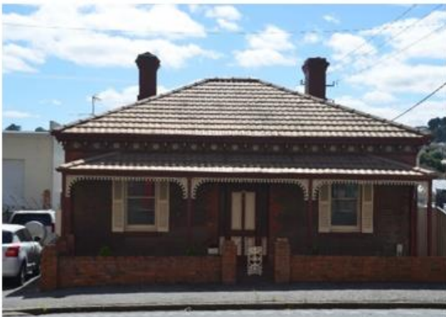
Figure 1 - Front façade, 25 Glen Dhu Street
