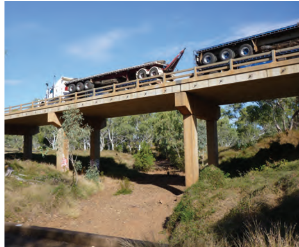
Bridge across the Cloncurry River Anabranch, mid 2012
