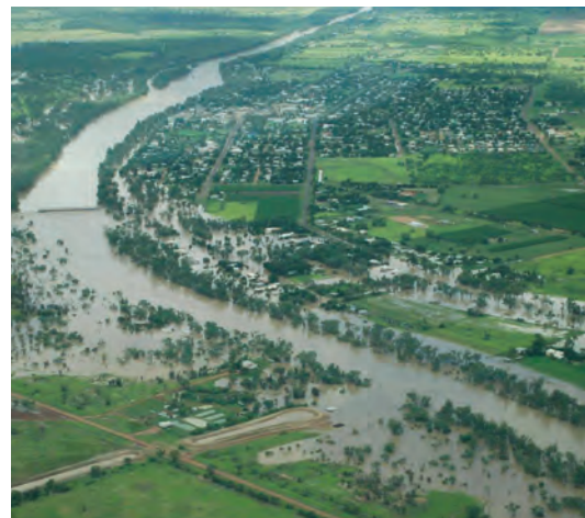
St George during flood in March 2010.
