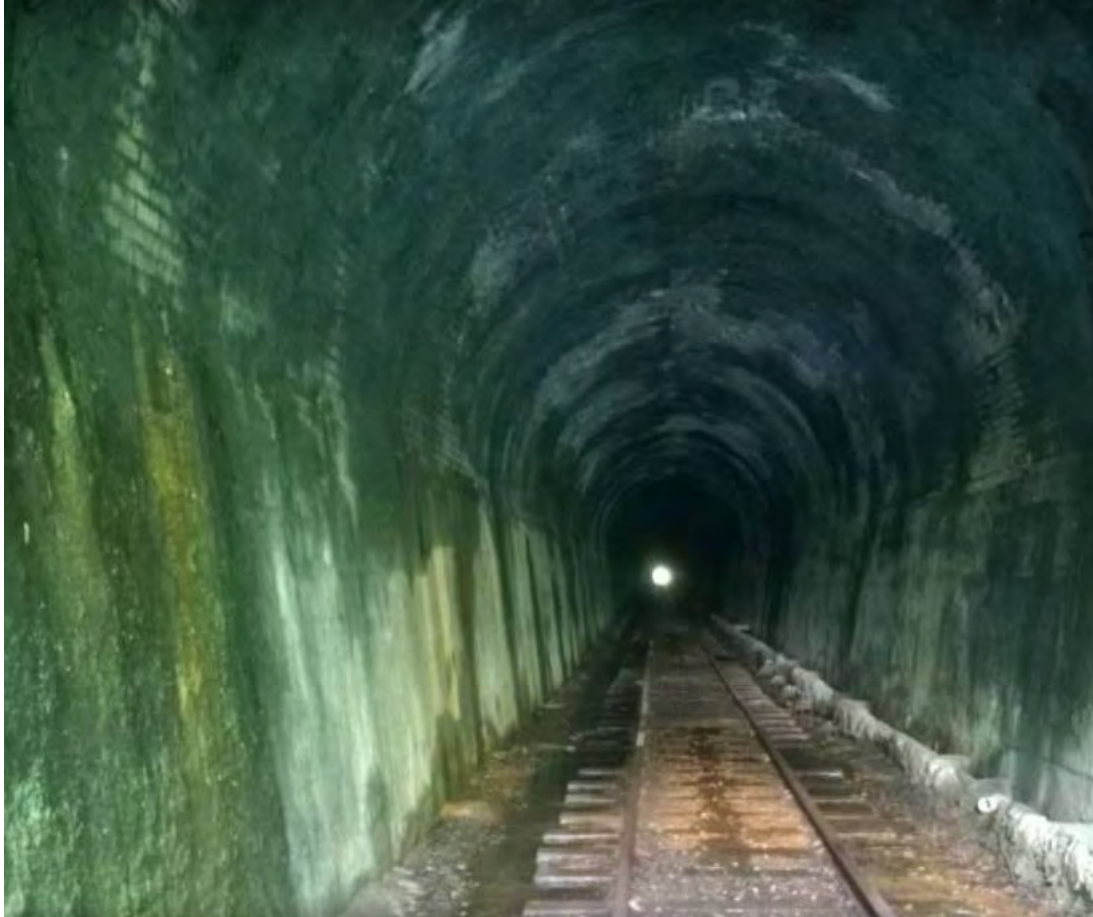
Figure 5. The long tunnel at Tunnel on the proposed trail extension
