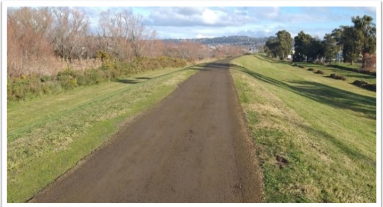
Invermay Levee Crest Rehabilitation with gravel, June 2020
