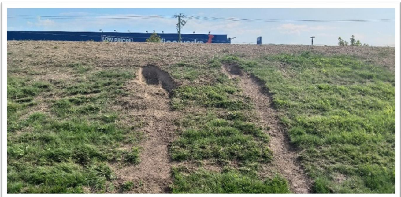
Four-wheel drive vehicle causing damage on flood levee in Tarooma St during winter 2020
