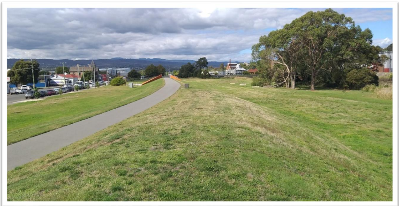
Low section on Invermay Levee for placing a temporary AquaDam to restore freeboard
