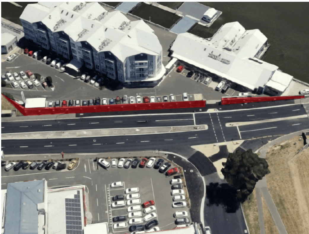
Figure 1 - Seaport levee wall (length of the proposed site)
