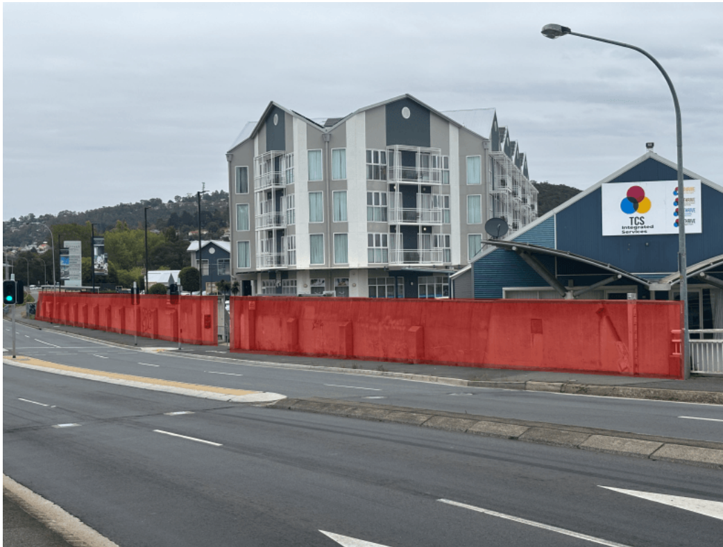
Figure 2 - Seaport levee wall (as seen from the footpath)
