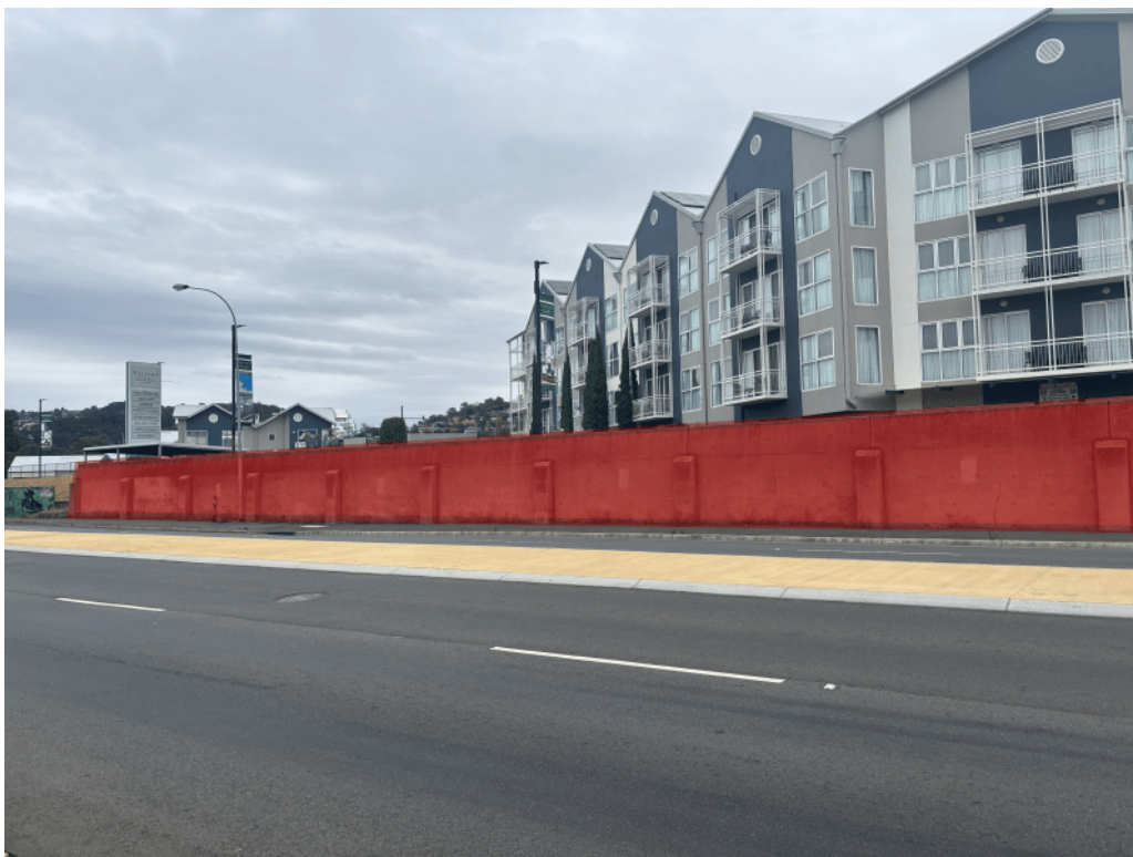
Figure 3 - Seaport levee wall (southern end)
