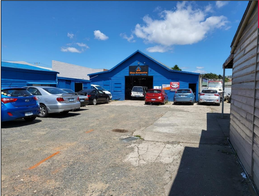
Figure 5: Mechanical workshop on site
