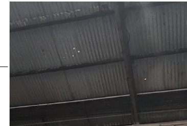
PATCH HOLES AND MAKE GOOD TO EXISTING CEILING
