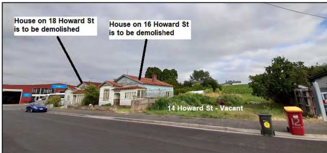
Figure 10: Looking North-west on to 14, 16 and 18 Howard Street
