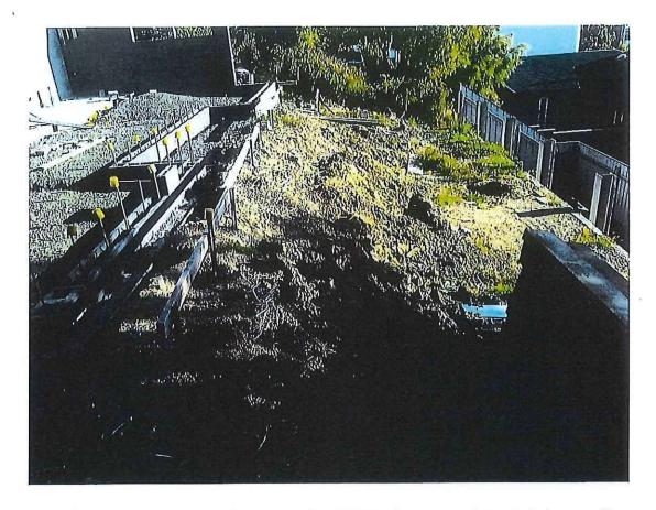
Another concern is that there is only 100mm between the retaining wall and the raised surface, which could be dangerous for anyone trying to walk along it but not wide enough for plants to be placed in the area. If the landowner wants a level area then perhaps stairs from the lower porch to the existing ground level would be more logical, as it would also give them the extra 100 mms.
