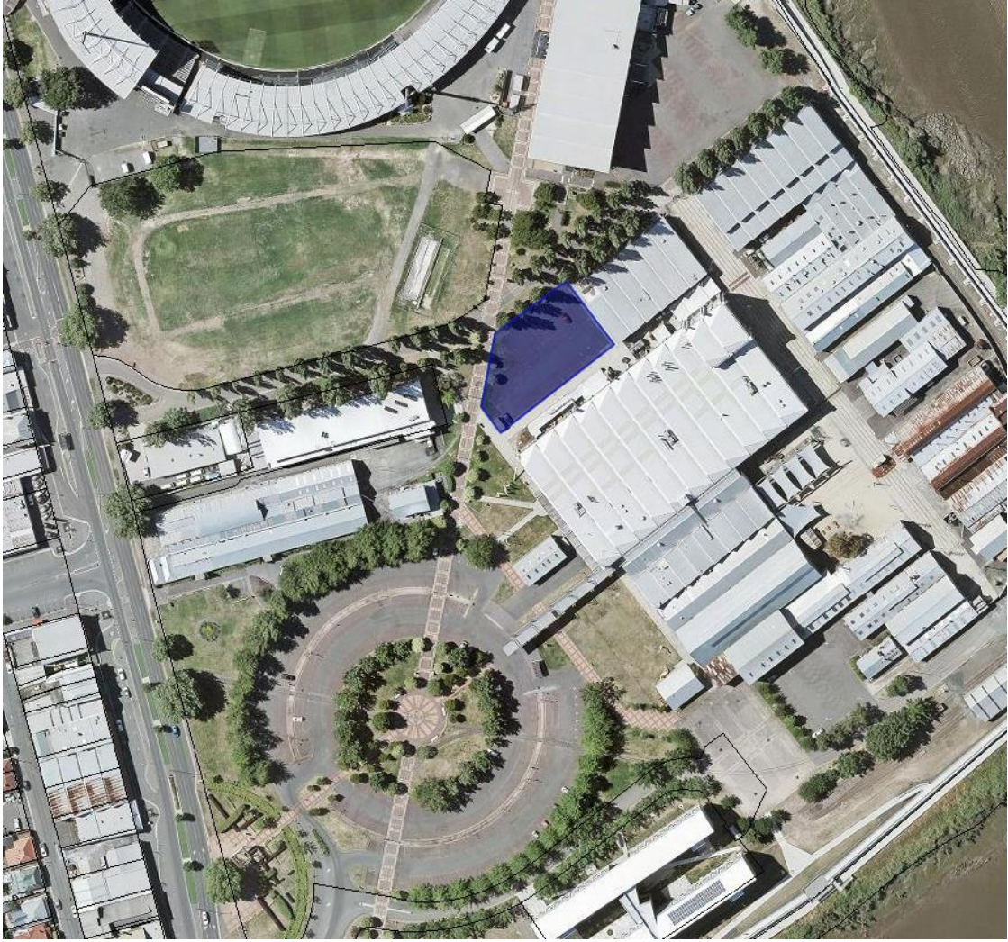
Figure 3: Aerial image with location of development site with aerial & cadastre (Source: www.theLIST.tas.gov.au )
