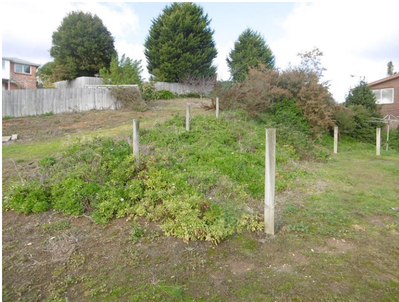
EXISTING EMBANKMENT COVERED IN LOW SHRUBBERY
