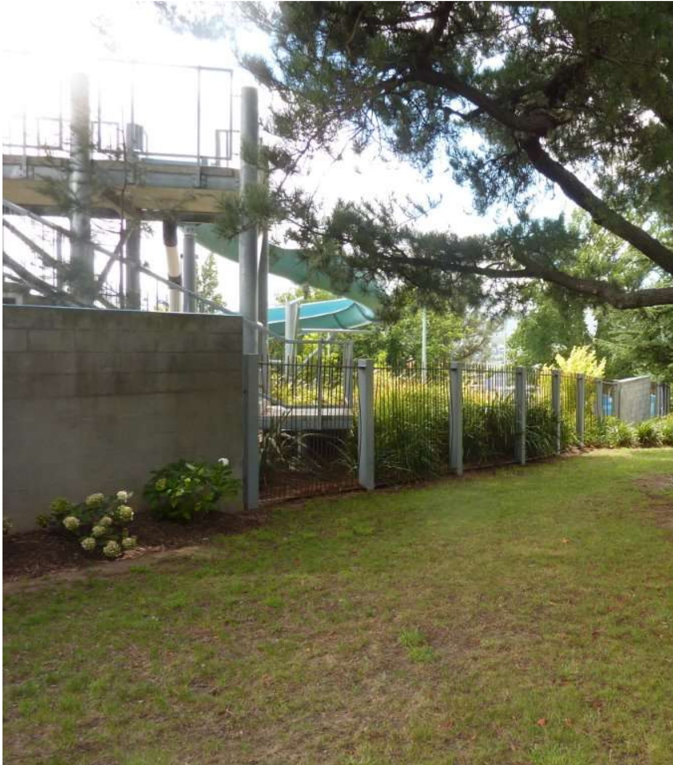
Photograph 2 Section of fence to be removed and replaced
