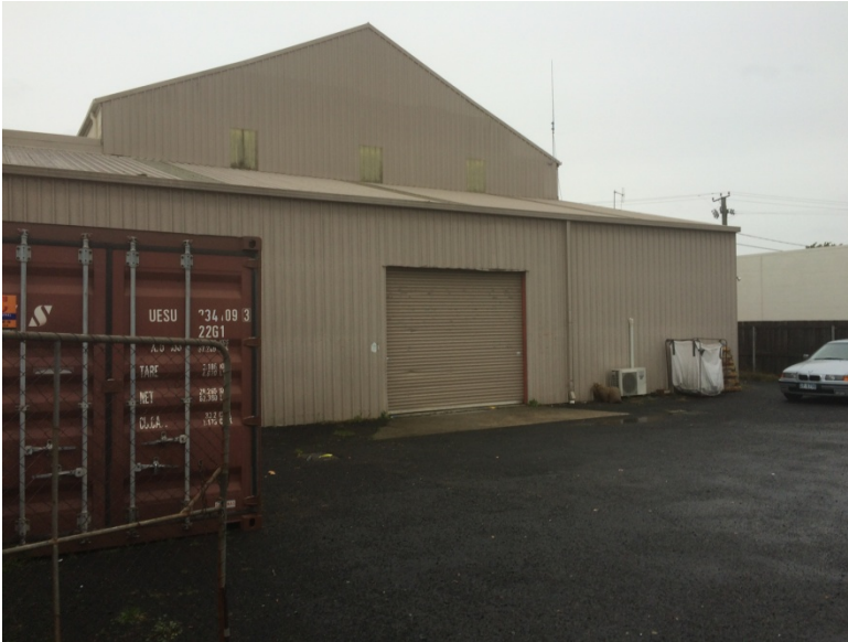
Figure 7 - Rear section to be removed and rebuilt in blockwork
