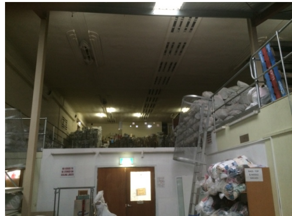
Figure 6 - The modern, low ceiling on the ground floor will be removed and this will expose the art deco ceiling above the dress circle (upper level).
