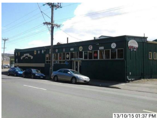
Automobile Museum Building (Cimitiere Street Frontage)
