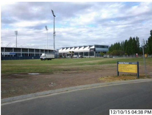
Southern boundary, north easterly aspect
