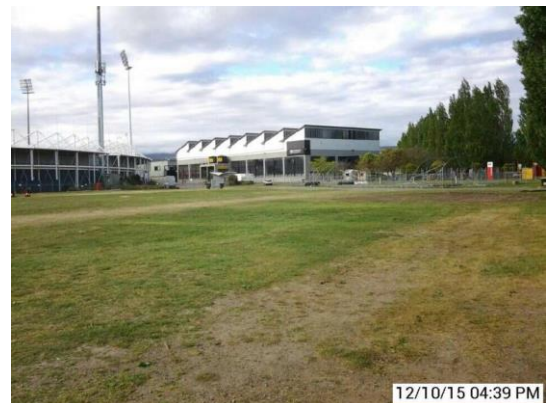
Rear area of site, north easterly aspect
