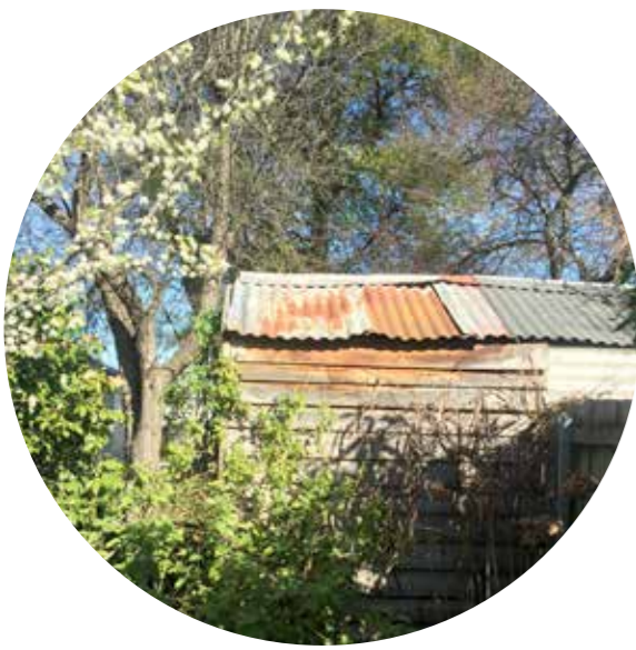
Existing out house rear
