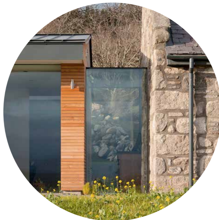
Glass threshold providing relief between existing & extension
