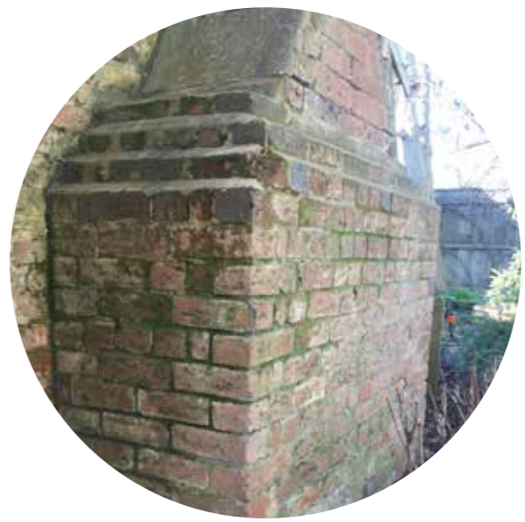
Existing brick chimney
