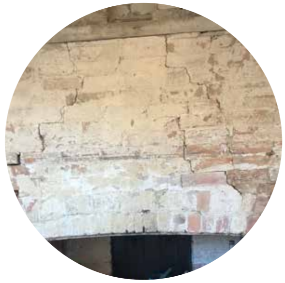
Existing end brick wall
