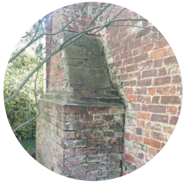
Existing brick chimney
