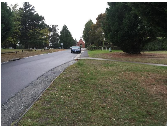
Fig 2.1 – Existing Road looking East to Finney Access
