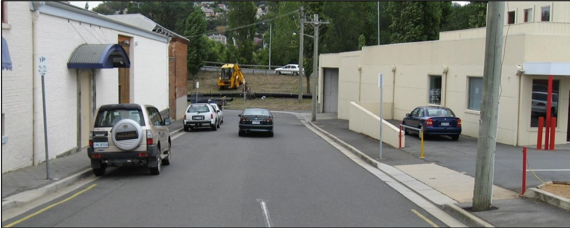
Figure 9: Canal Street, looking west along the site's northern boundary
