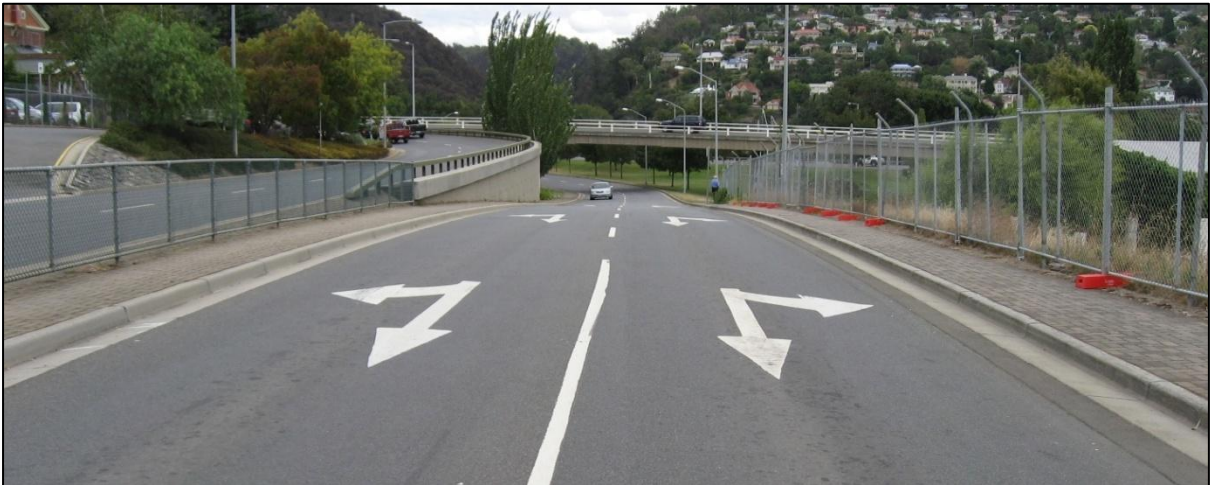
Figure 5: Cimitiere Street, looking north-east at the intersection with Charles Street
