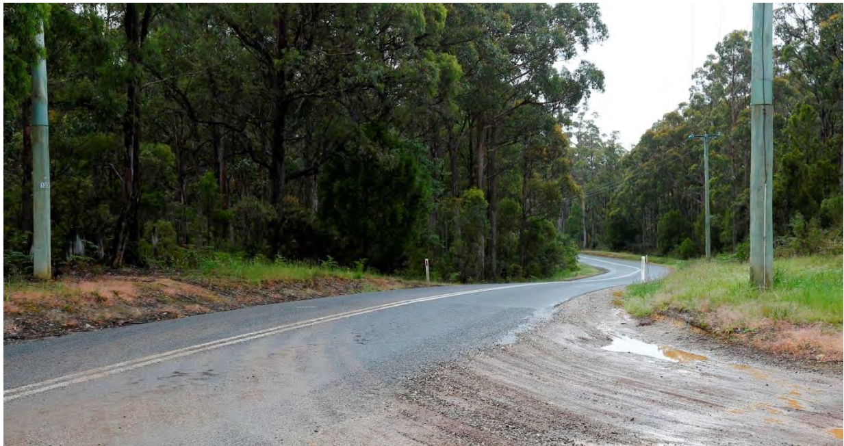
Figure 3 Pipers River Road junction with Colgraves Road
