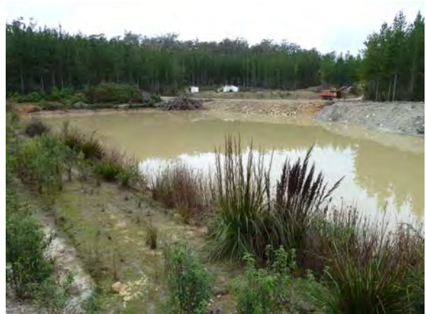
D. Existing sediment settling dam
