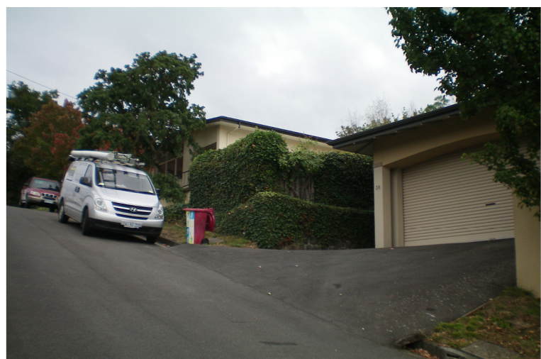
SHOWING ELEVATED POSITION OF 40 ANN ST
