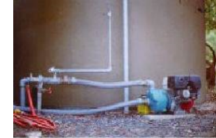
Protect above ground pipes and pumps
