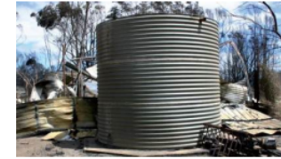
Colorbond non-combustible steel tank
