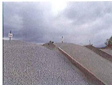
Concrete aggregate bins water spray system to reduce the effect of wind blown dust
