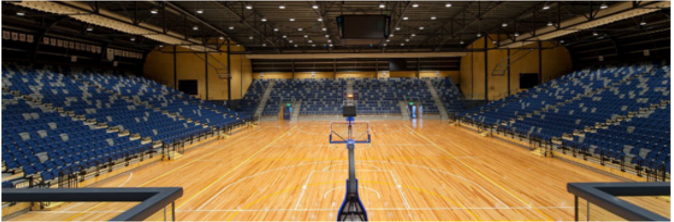
The recently constructed Bendigo Stadium
